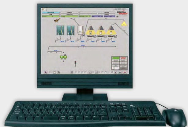
Operator supervision station
