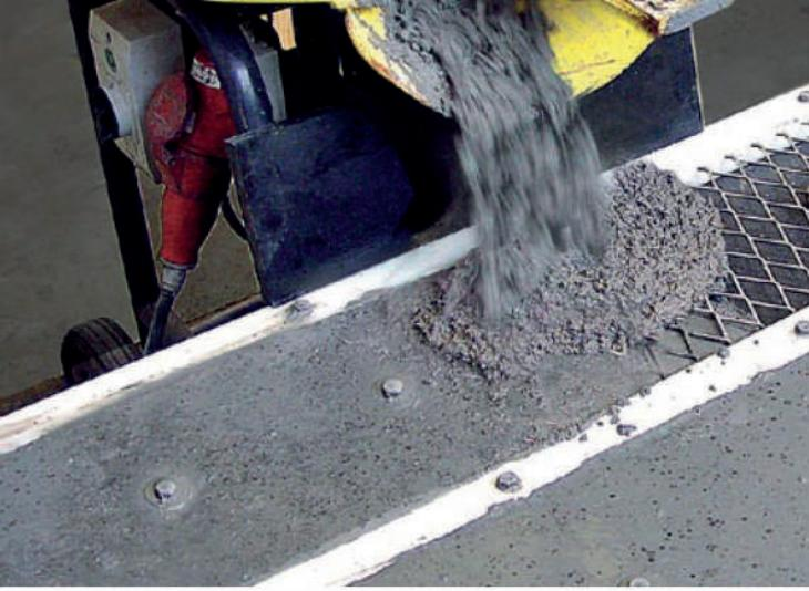
Refractory castables (concretes) are compressed as dry compounds containing alumina cement with aggregates: chamotte , bauxite, alumina, etc.
