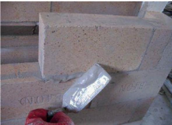
Refractory and insulating mortars are composed of powders of very fine powders refractory materials mixed with adhesive refractory soils and are used to stick refractory and insulating bricks. Mortars are heat-set.
